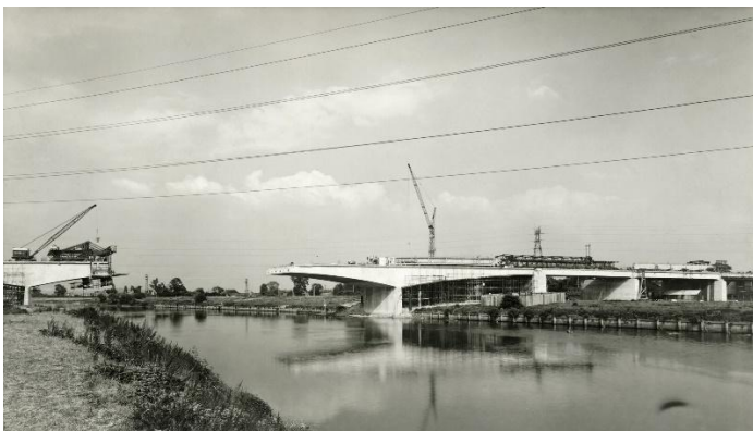
First bridge under construction 1957....
