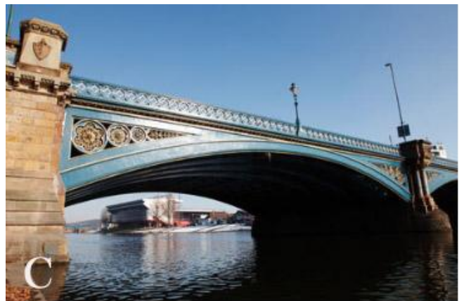
Copied photo as repair work currently obscures much of the bridge.
