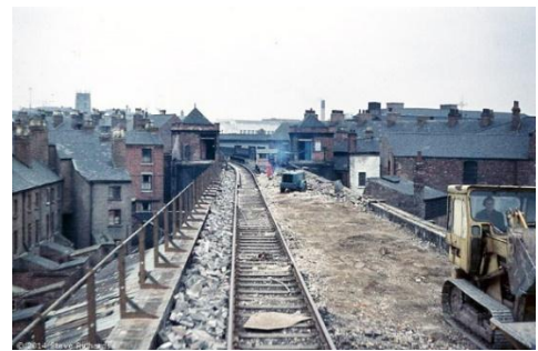
Arkwright Street station (being demolished, the platforms already removed).
