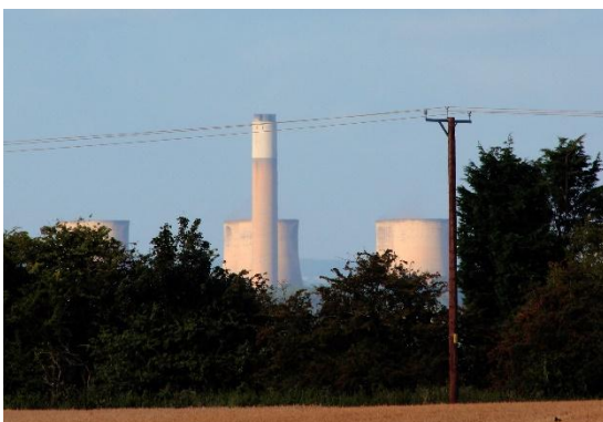
Ratcliffe Power Station
