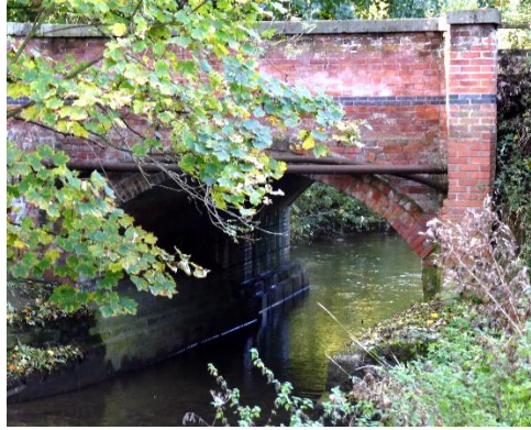
...looking back – the bridge over the Brook
